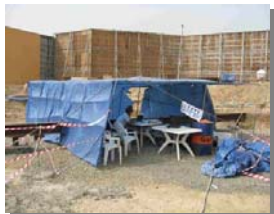
Testing in progress sheltered from the elements
