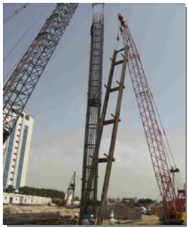
Lifting of O-cell assembly prior to installation
