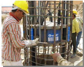
Installation of one of the O-cell assemblies
